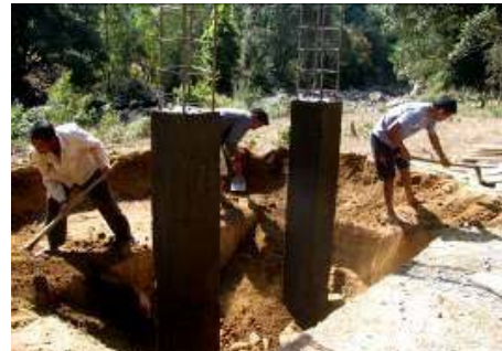
Figure XVIII: Bridge construction in Mandalgre
