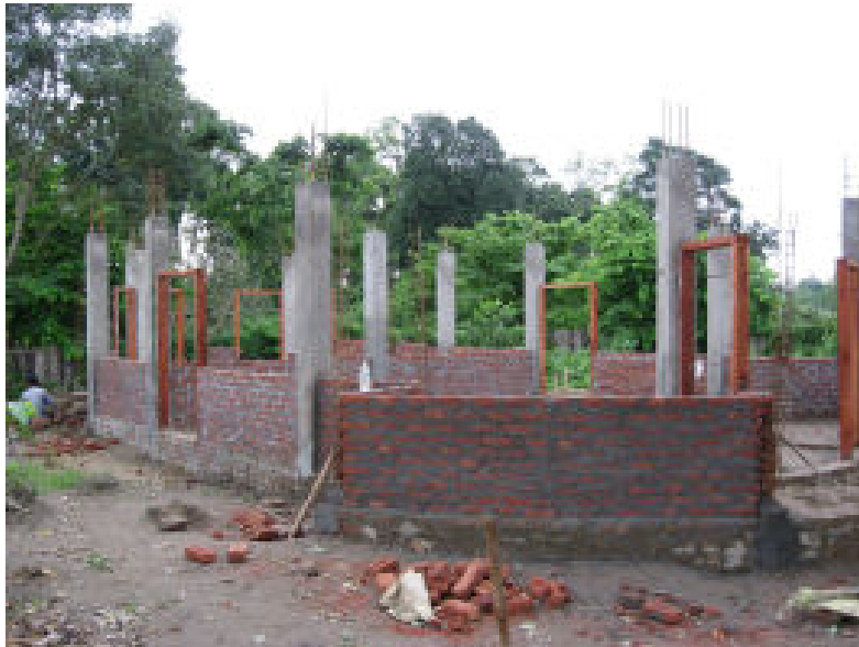
Office and retiring rooms under construction at CWRC
