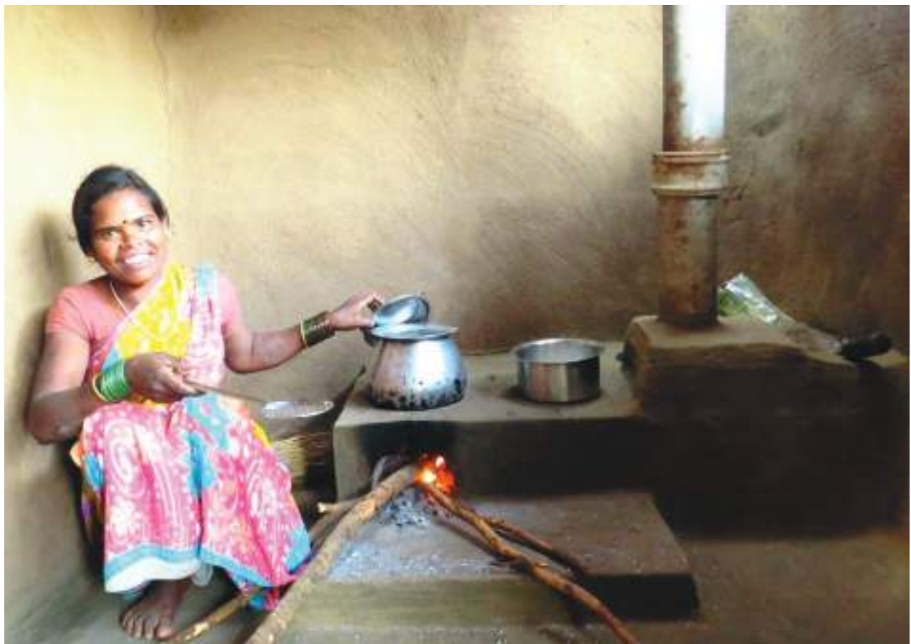
Fig 5.14 Improved Cook Stove installed in USTR villages to reduce fuelwood usage and improve health of women folks.
